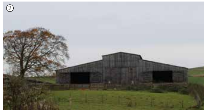
▲ Large storage Barn
