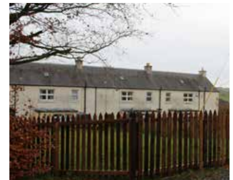
▲ 3. Properties along eastern access track
