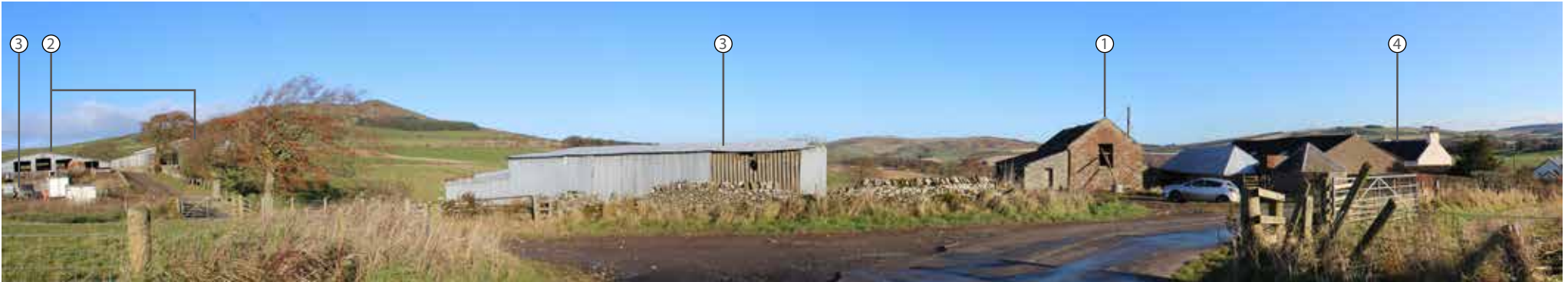
▲ Existing stone barn and auxiliary buildings
