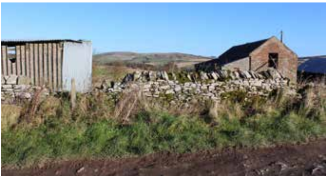
▲ Dry stone wall
