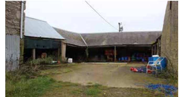
▲ Existing storage shelter
